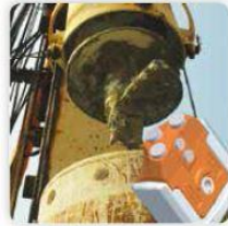
5 - Foundation drilling
