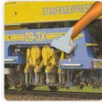
14 - Rail track construction
