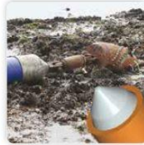
7 - Horizontal directional drilling HDD
