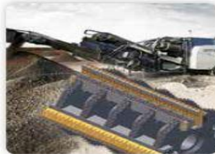
6 - Crushing and mixing
