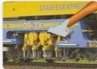
14 - Rail track construction
